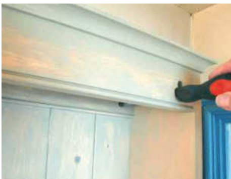
STEP 23. Support the unit and mark wall for fixing, checking for level. Drill and insert plugs for screws
